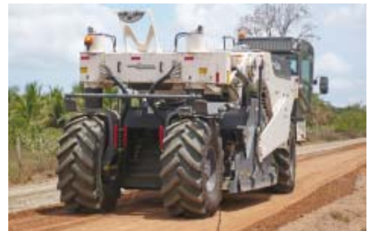
Base recycling on SE-204, on the Tatú stretch in Pacatuba
