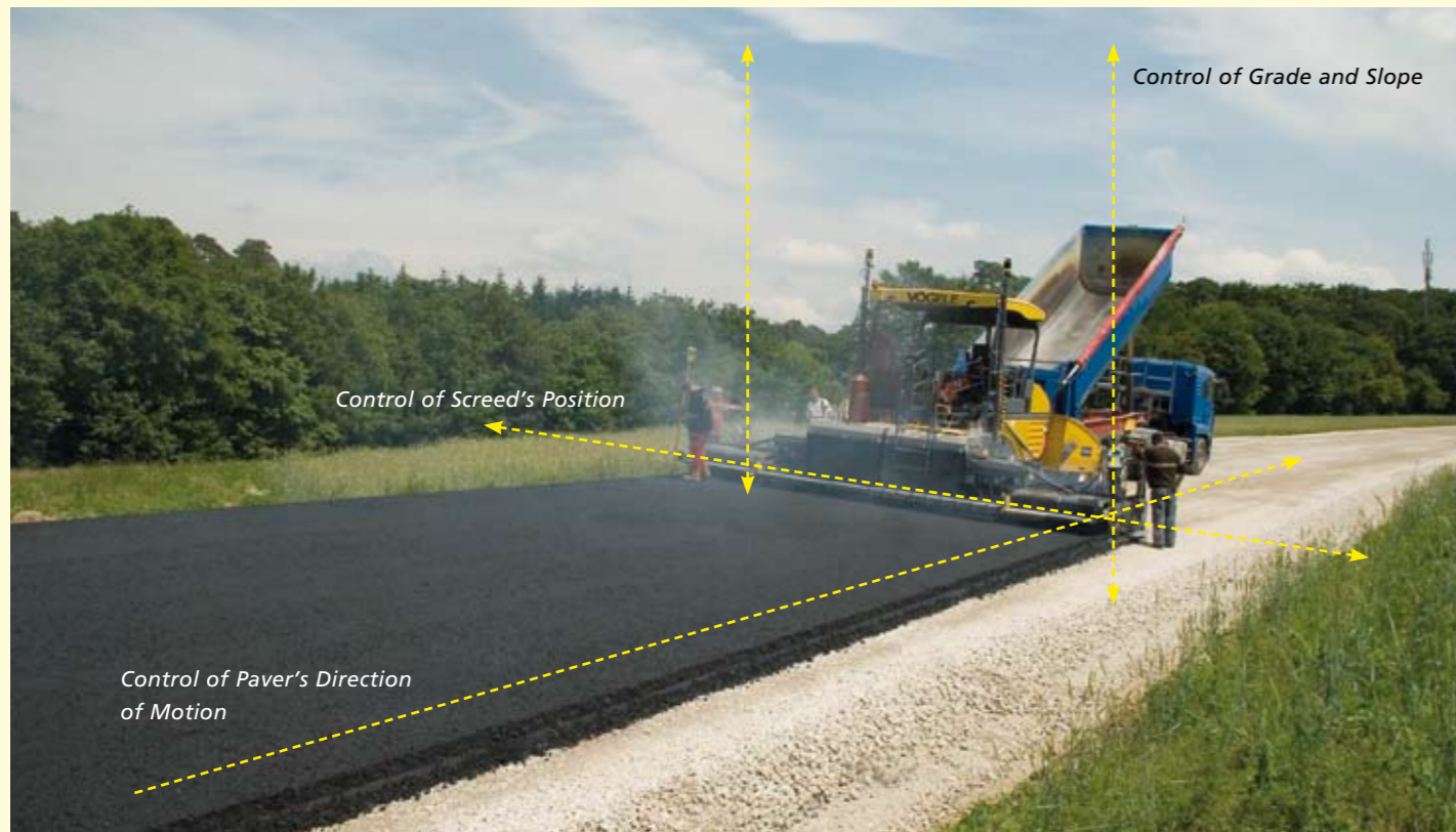
NAVITRONIC® Plus controls the screed's position fully automatically.
