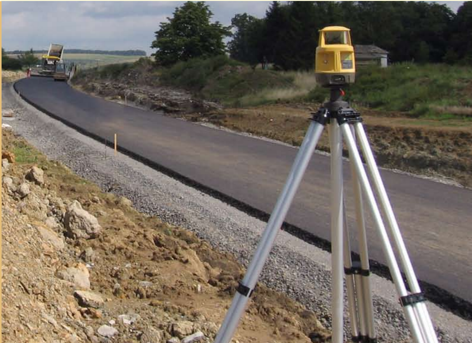
Accurate control of the screed width by NAVITRONIC® Plus guarantees a screed position in absolute compliance with the route's design. No matter whether steering is manual or automatic.
