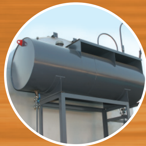
Integrated Diesel Tank
